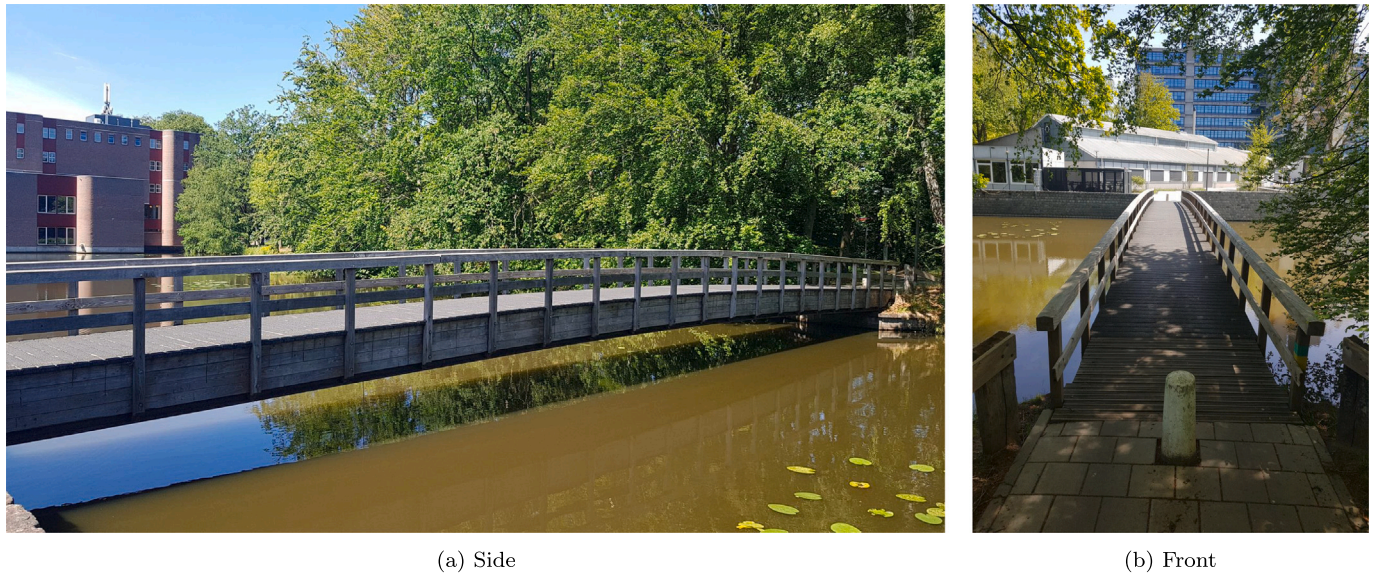
Fig. 2. Photos of the UT campus footbridge.
